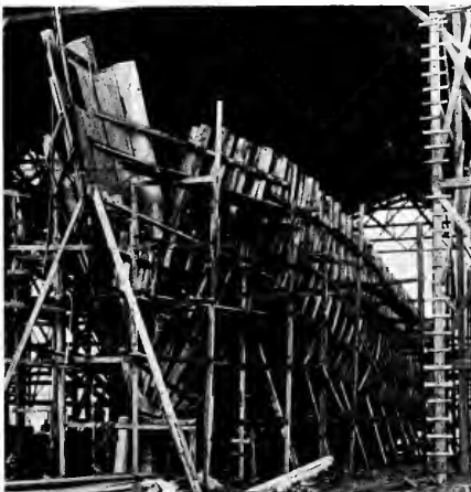
Bow view of vessel No. 1 at the Columbia Engineering Works.
